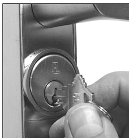
Fig. 1b: Center keyway toward bottom
