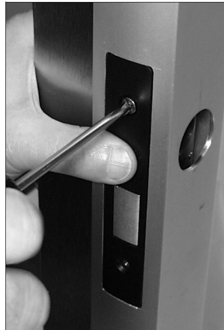
Fig. 4d: Install the deadbolt face plate
