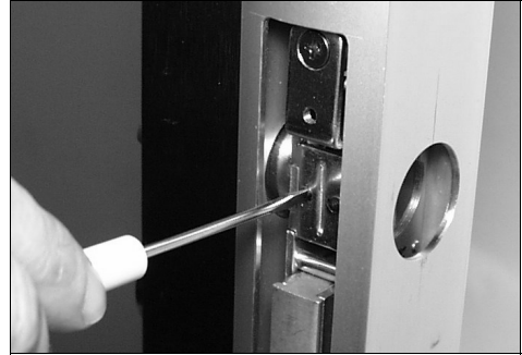
Fig. 4c: Secure interface cylinder to lock
